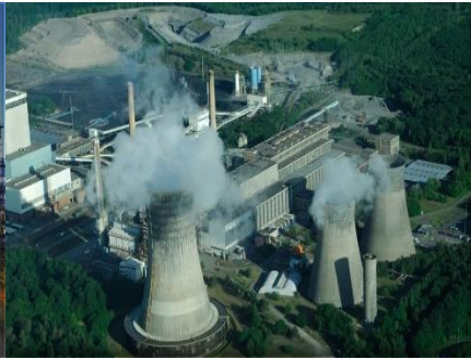
Electricity generation, coal and gas-fired power plants
